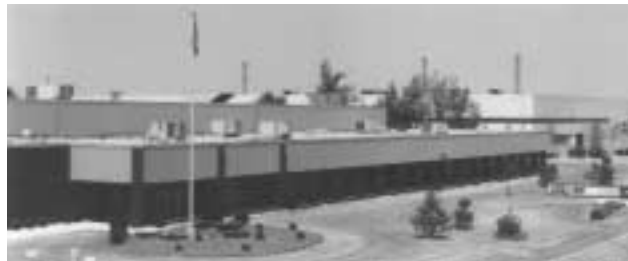
QSS plant in Tecumseh, Ontario.
